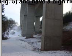
Fig. 4: Viaduct A 60: safe crossing possibility
