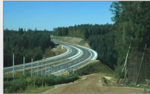
Fig.1: A 60 with wildcat-proof fence in the construction phase
